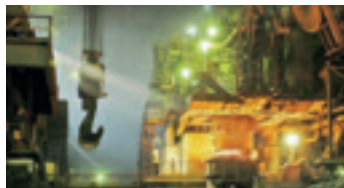
1959: Continuous casting machine
